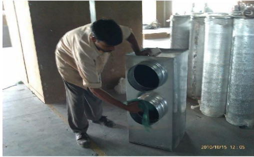
Cleaning Prior To Installation
