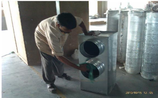
Cleaning Prior To Installation
