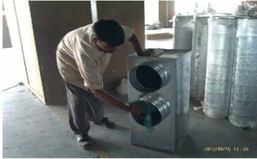
Cleaning Prior To Installation
