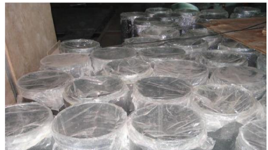
Ducts Stored with Properly Wrapped with plastic
