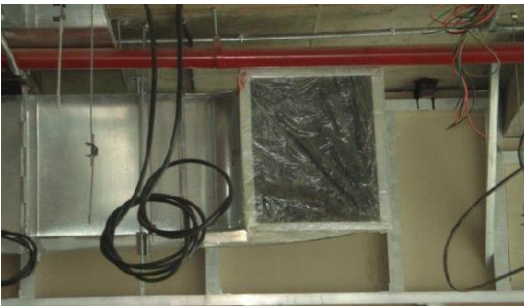
Ducts Wrapped With Plastic To Avoid Dust Cleaning Prior To Installation
