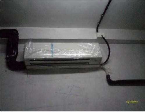
Equipment covered during Construction Phase
