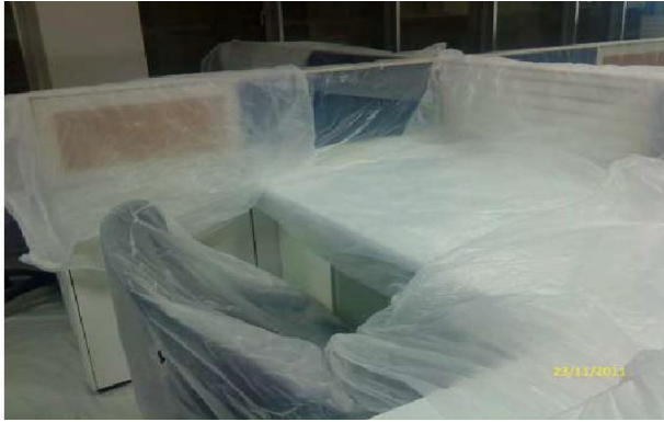
Equipment covered during Construction
