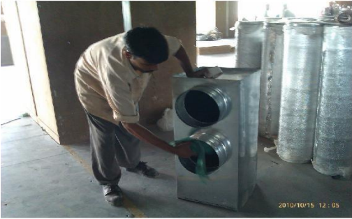
Cleaning Prior To Installation
