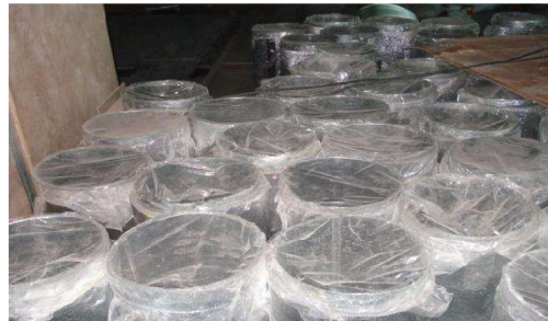
Ducts Stored with Properly Wrapped with
