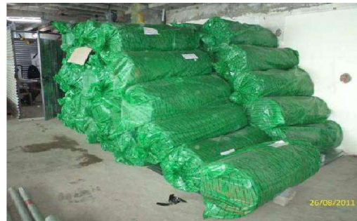
Ducts Stored with Properly Wrapped with
