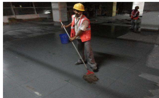
Cleaning of Site on regular basis
